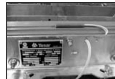
Fig. 4 1 or 2 PT100 on the core
